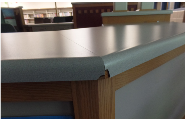
SAWYER - Millwork damage
