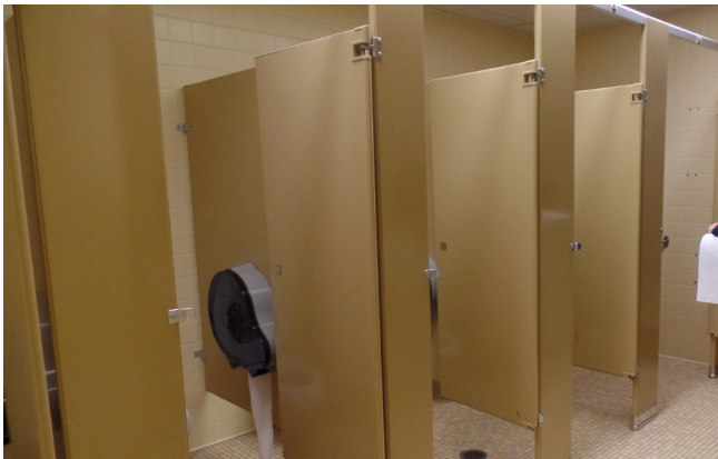
SUNSET - Inaccessible restrooms (ADA)
