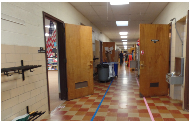
SUNSET - Asbestos floor tile
