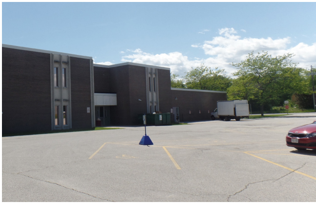
HIGH SCHOOL - Accessible (ADA) parking and loading zone not properly marked / identified
